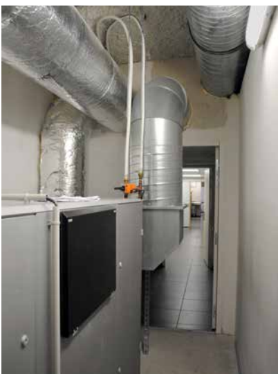
Installation double-flux © CAUE 14
